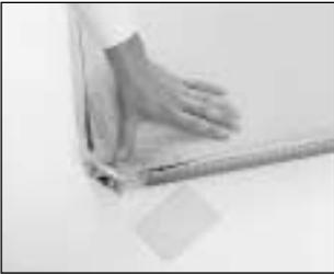
While applying pressure on fabric between rollers at corner section, press down on locking strip or rods using rigid scraper. Be sure mesh/line comes in at an angle.
