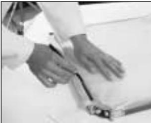
Use alignment grooves in roller to make adjustment line. If roller does not have alignment grooves, use locking strip channel.
